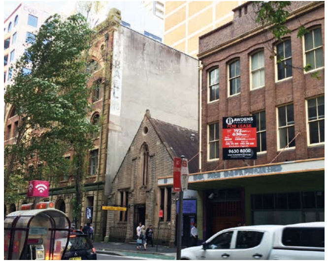
E_32 York Street SCA - Kent Street 420 Kent St Heritage Item
